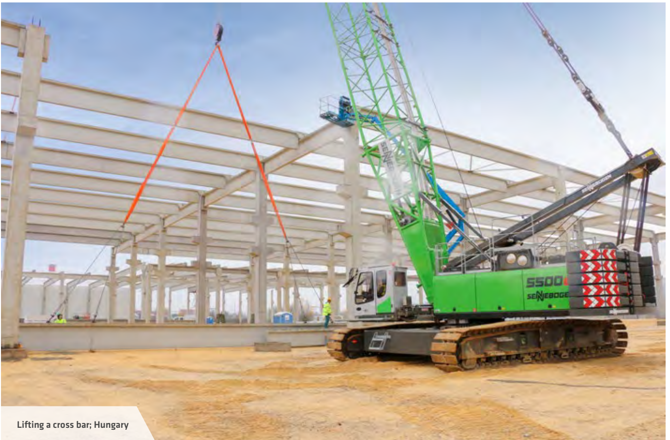
Prefabricated component assembly; Germany
