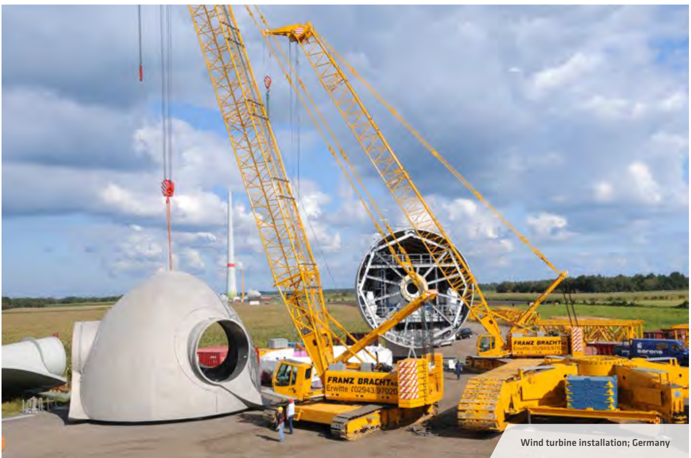
Prefabricated component assembly; Germany
